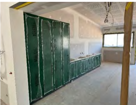
Inside one of the Prep-2 classrooms, not yet completed
